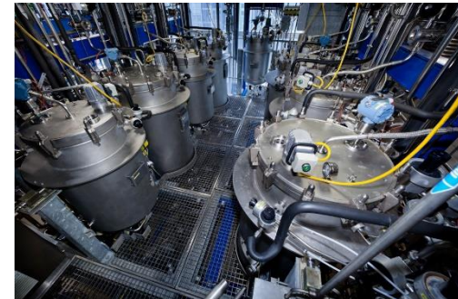
Feed vessels of fermentation department
